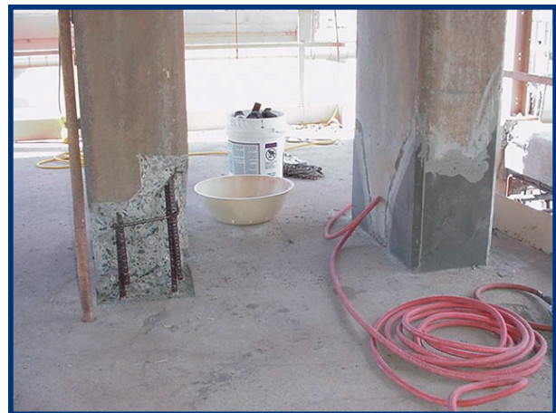
Columns before and after repairs
