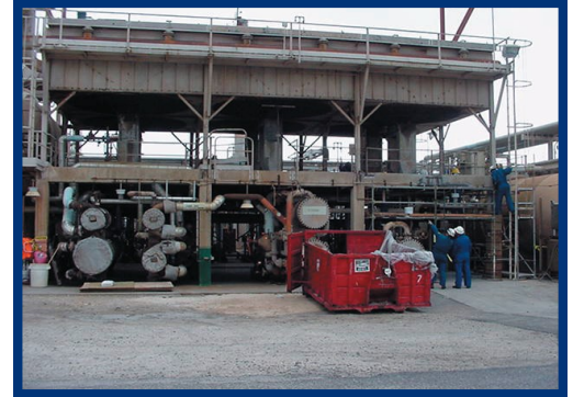
Fin/Fan structure in Hawaii
