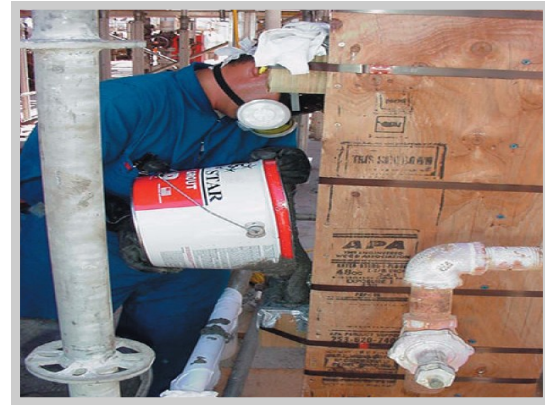
Pouring columns with Five Star DP Epoxy Grout
