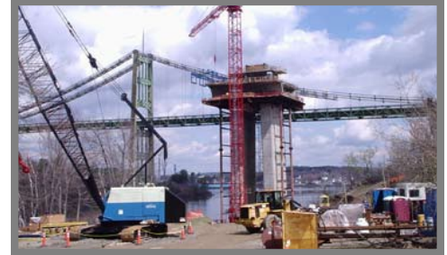
Penobscot Narrows job site—Maine
