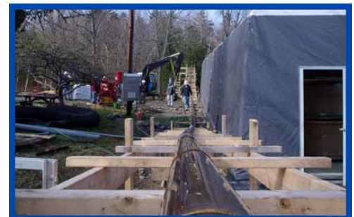
Field testing of Five Star® Special Grout 400
