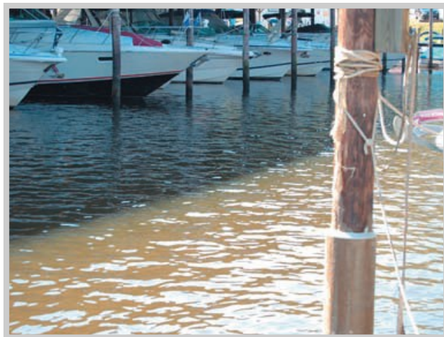
Completed pile jacket rehabilitation with jacket in place
