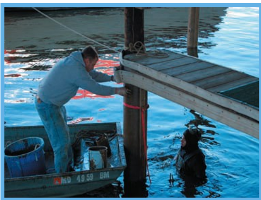
Hand capping the pile to finish the rehabilitation
