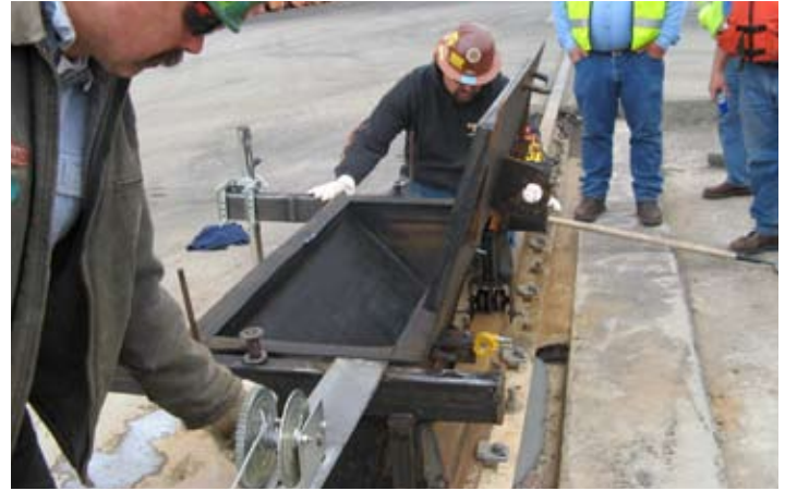
Mobile headbox designed for pouring HP Epoxy Grout
