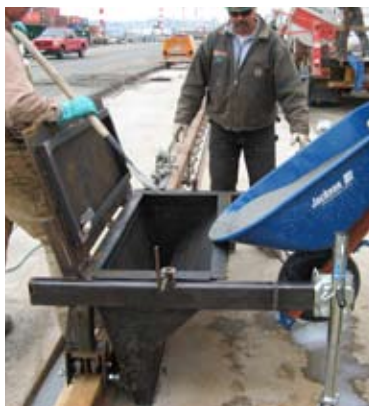
Pouring Five Star® HP Epoxy Grout in mobile headbox
