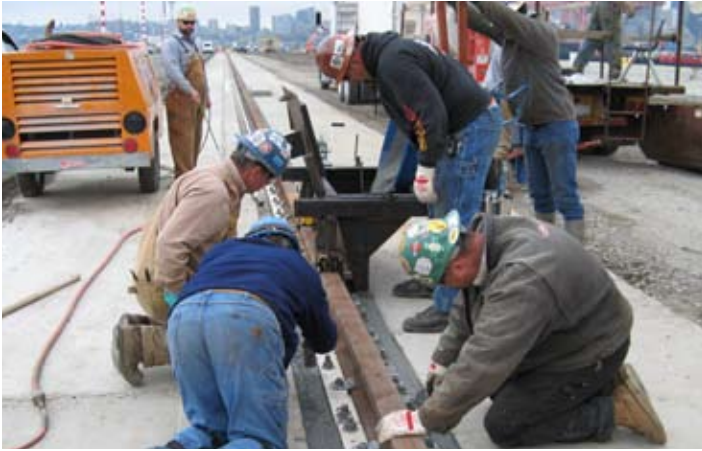
Grouting of crane rail
