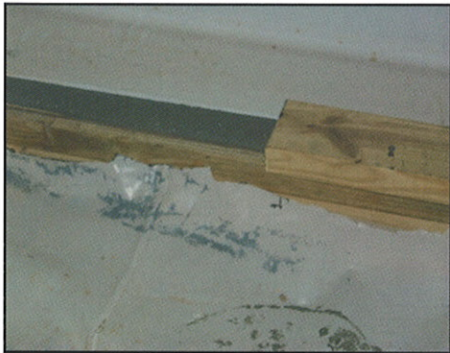
Completed Pour After Flowing 14 Feet
