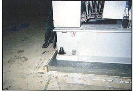
Finished Chamfered Edge After Removing Form
