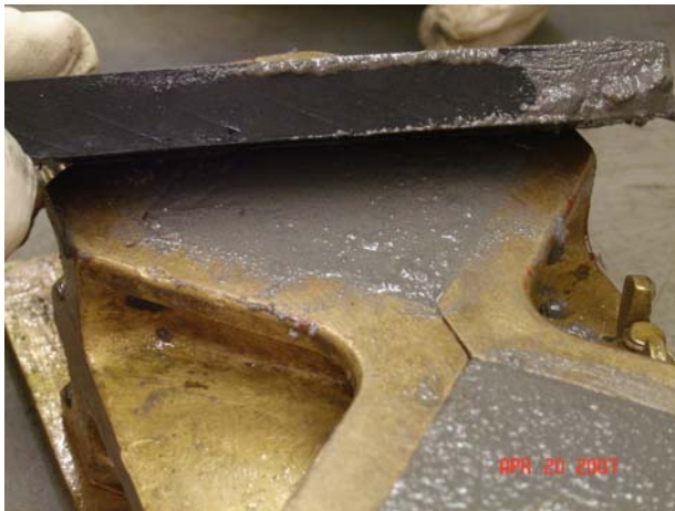
Screed off excess epoxy grout using a trowel or tongue depressor and clean off any excess material on top of the mold.
