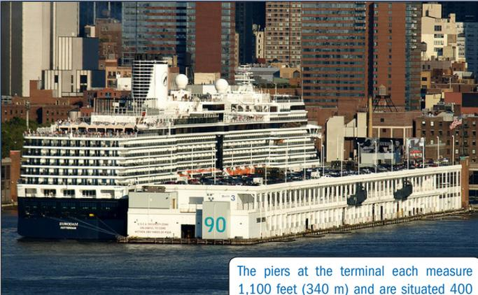
The piers at the terminal each measure 1,100 feet (340 m) and are situated 400 feet (120 m) apart; each pier is supported by roughly 1,500 untreated Douglas Fir timber piles, and concrete pedestals support a 10-inch (25 cm) reinforced concrete deck and the superstructure columns of the two-story steel-framed terminal building with roof parking deck.
