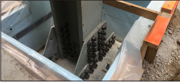
Preparation Includes Creating Forms Around the Beams
