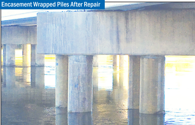
Encasement Wrapped Piles After Repair
