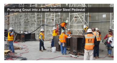
located in the center of the formwork the grout had to flow around. All of this combined with an increased minimum strength requirement of 13,000 psi and roughly 6 cubic feet of grout. Both joints required a 95% EBA minimum with no void larger than 1 square inch. Each joint would be disassembled and inspected for compliance throughout the duration of the project.
