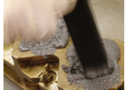
D.3. Fill molds with second layer of epoxy grout, then consolidate to remove entrapped air.
