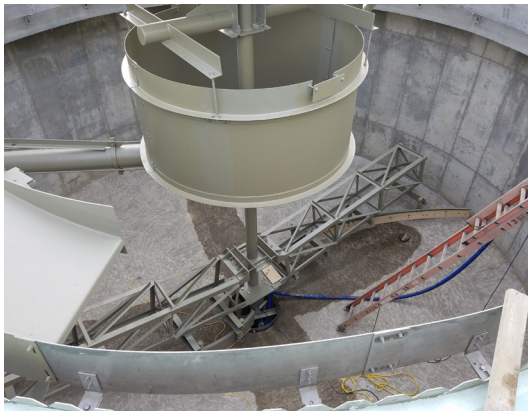
A CLARIFIER TANK PRIOR TO INSTALLING GROUT.
