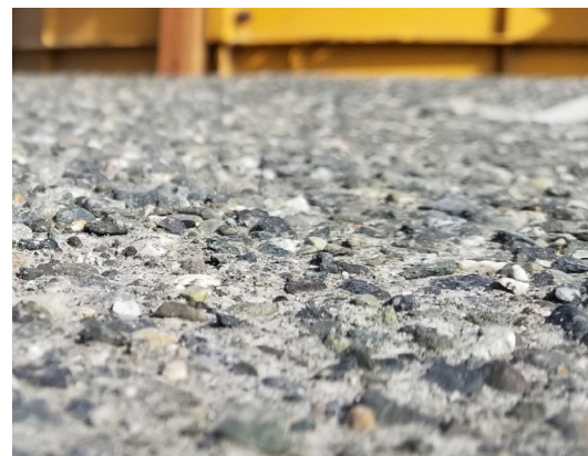
SURFACE PREPARATION USING A "SURFACE RETARDER". ADDITIONAL SURFACE PREP MAY BE REQUIRED TO ACHIEVE CSP10.
