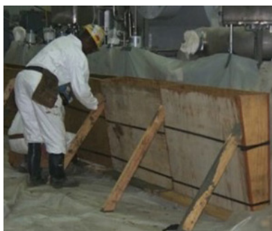
ON LARGE PLACEMENTS, MULTIPLE HEADBOXES ARE OFTEN EMPLOYED. THE GROUT IN THE PHOTO ABOVE PROBABLY NEEDS TO FLOW 6-8 FEET (1.8 - 2.4 M.).
