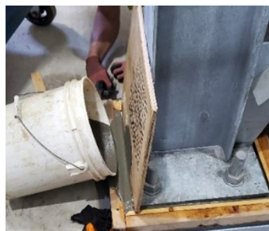
ON SMALL APPLICATIONS A HEADBOX CAN BE AS WIDE AS THE PLATE SO IT DOES NOT NEED TO BE MOVED. ALSO IT CAN CONTROL THE GROUT AND SPEED UP THE GROUT FLOW.
