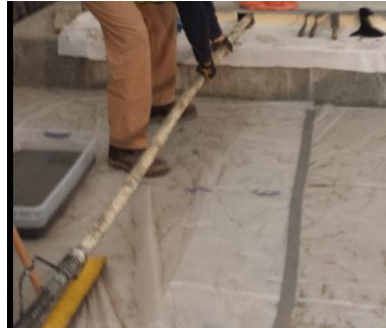
OTHER METHODS INCLUDE USING LONG PVC NOZZLES TO TRANSPORT THE GROUT.
