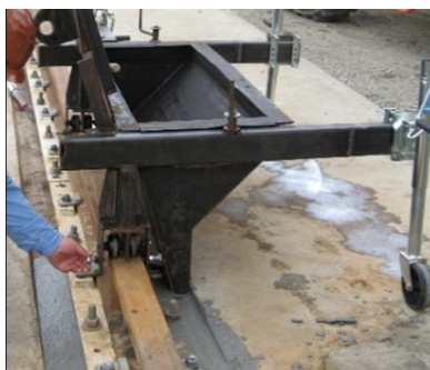
ON LARGER REPETITIVE GROUT INSTALLATIONS MULTIPLE OR SPECIALIZED HEADBOXES MAY BE CONSTRUCTED TO EXPEDITE THE PLACEMENT PROCESS.
