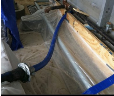
“LAY FLAT” HOSE IS OFTEN USED TO TRANSPORT GROUT TO THE FAR END OF THE FORMS UNDER EQUIPMENT. THE HOSE IS EASY TO INSTALL AND IS “PULLED BACK” AS THE GROUT IS PUMPED.
