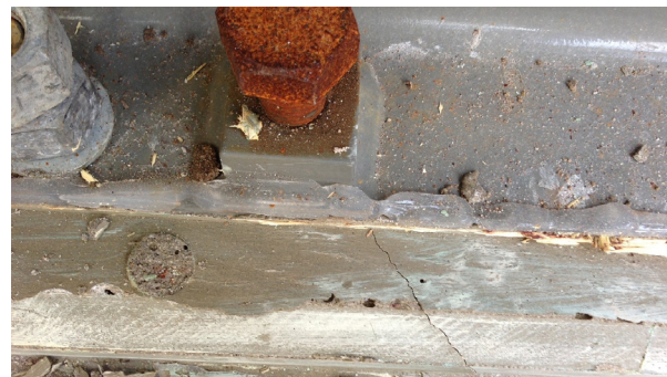
VERTICAL CRACKING OFF A JACK BOLT
