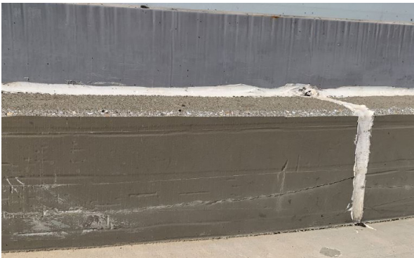
VERTICAL CRACK REPAIR IN EPOXY GROUT USING ELASTOMERIC JOINT SEALER
