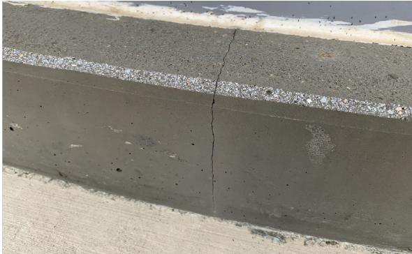
VERTICAL CRACK IN EPOXY GROUT
