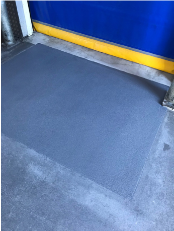
RSR Easy Mix™ prior to epoxy coating.
