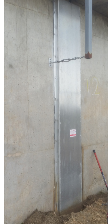
Joint sealant system installed over Five Star Structural Concrete® V/O.
